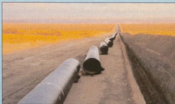
Pipe ready for welding in the deserts of Dubai
